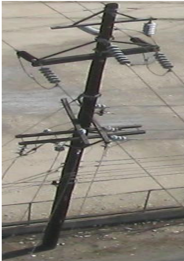
Figure 4: Photo of Faulted Pole Structure #1 on the Duhaney to Naggo Head 69kV Line
