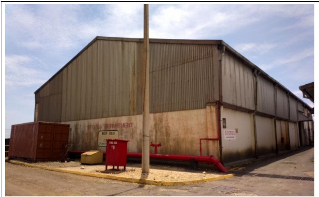
Photo 2 – Main Stores Building ( Concrete and metal sheeting)
