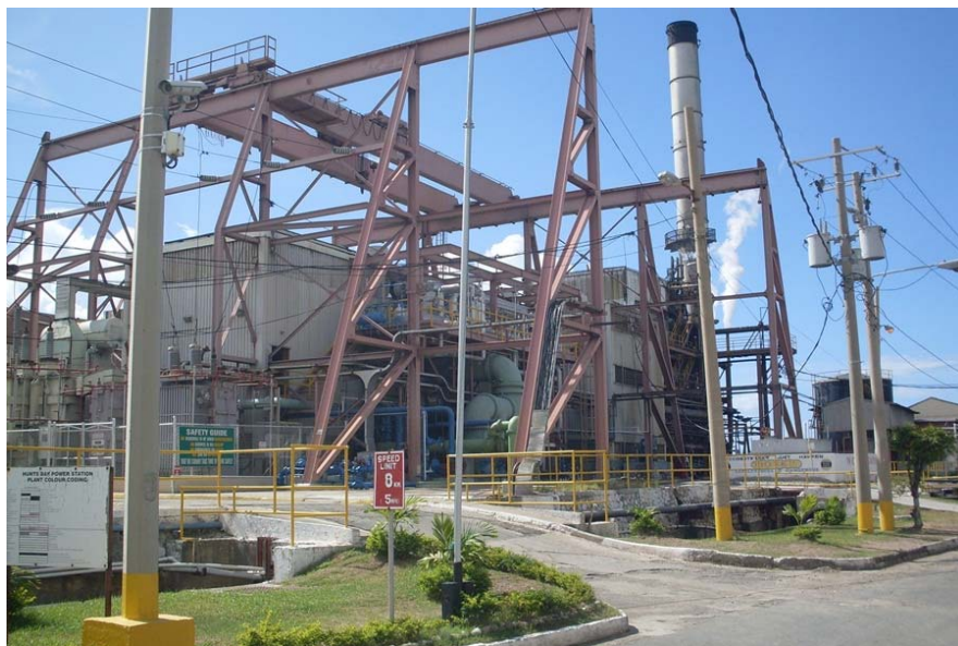
Photo 1 – Hunts Bay Power Plant Unit B6 – Crane Structure
