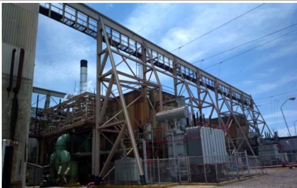
Photo 5 - Northern end of plant/crane structure
