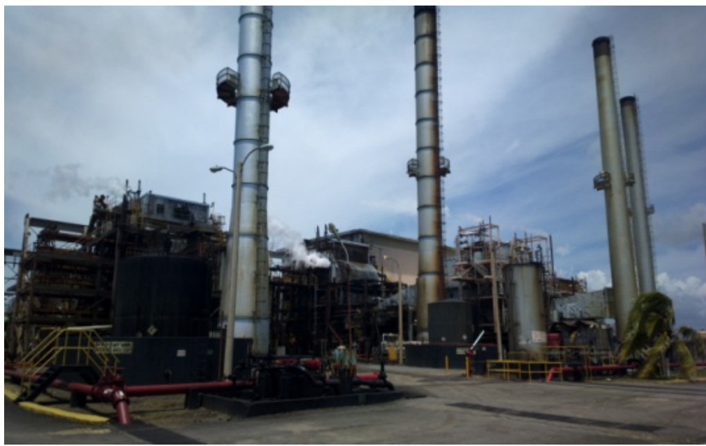
Photo 4 - Southern End of Plant Stack
