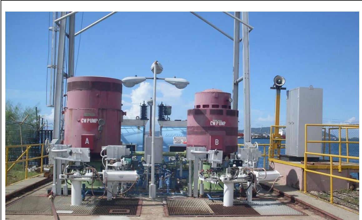
Photo 2 – Hunts Bay Unit B6 Intake
