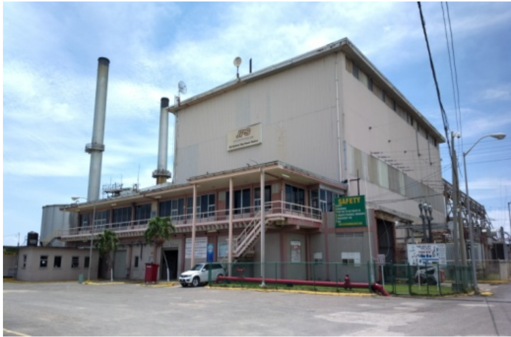
Photo 1 – Old Harbour Plant front and Admin. Building
