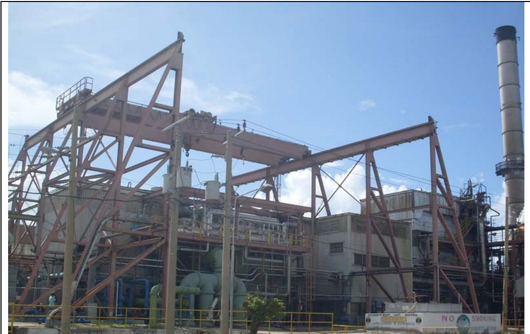
Photo 5 – Hunts Bay B6 – Crane Structure
