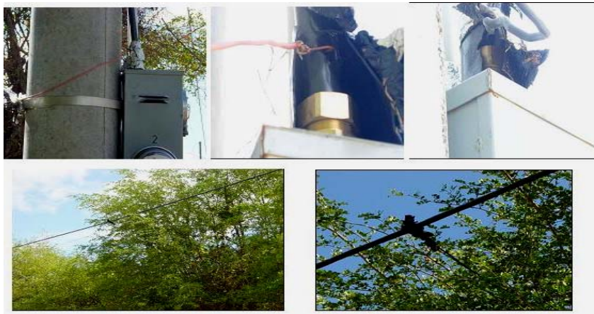
Figure 9.8: Evidence of Network Tampering
