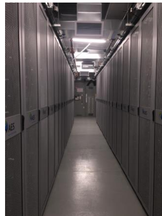
DPP, Battery Enclosure Interior
