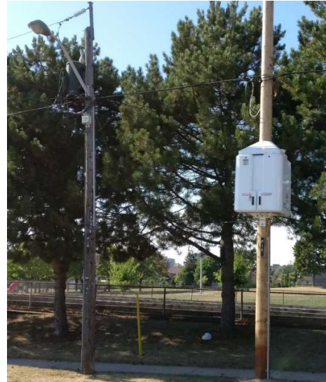
Distributed Generation Energy Storage
