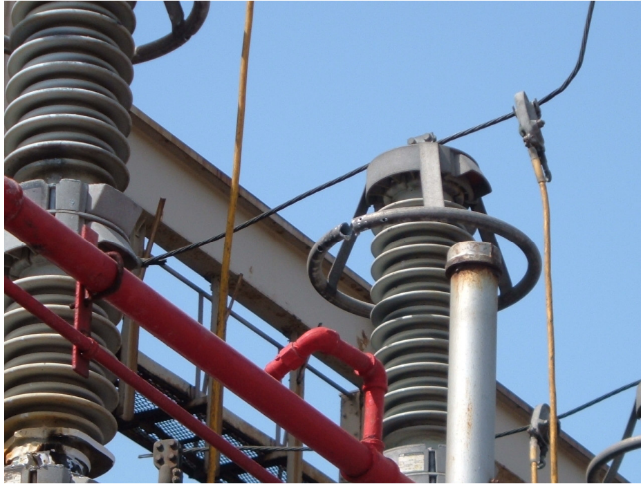
Photo #4: Burn-through of corona ring at top of arrester – middle phase
