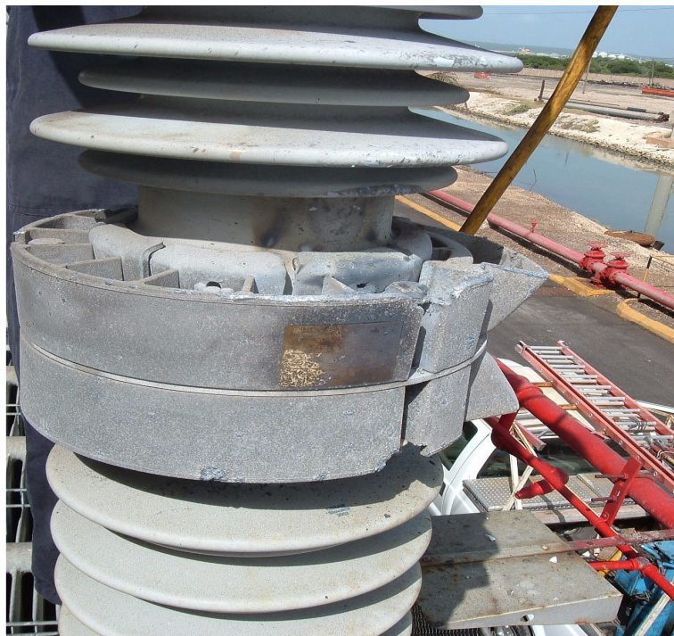
Photo # 3: Scorching on middle phase arrester
