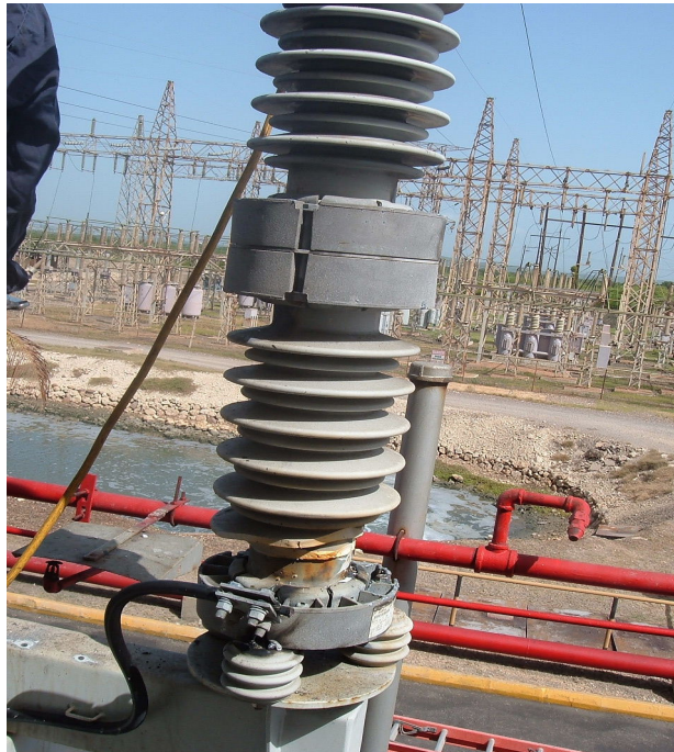
Photo #1: Burnt ground conductor connector at base of outer phase arrester
