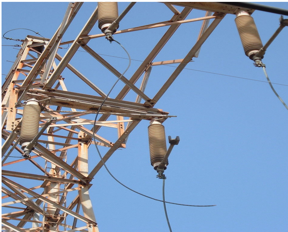
Photo #5: Dislodged down dropper on middle phase of disconnect switch 9-227
